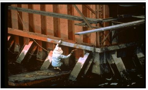
Airless spray equipment was used to apply Epodur®2755 urethane-modified epoxy primer to steelwork in the seaward corner of the coal-unloading pier. The corrosion-inhibitive primer is very tolerant of surface moisture, cures more quickly and at lower temperatures than conventional polyamide-epoxy primers, and provides excellent adhesion even in severely corrosive environments and in continuous immersion service.
