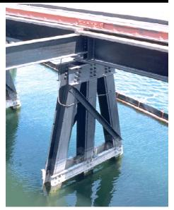
Comprehensive protection of steelwork in dock and coal unloading area ia assured by use of Epodur 2755/Epodur 782 coating system in conjunction with cathodic protection. Intercoat adhesion to sound, previously applied coal tarenamel coating is excellent, and the coatings have proven to be resistant to cathodic disbondment and the effects of tides and winter ice.
